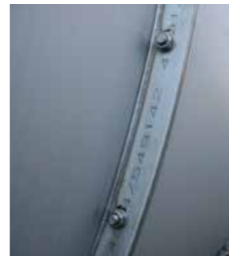
Stainless steel flange connection
