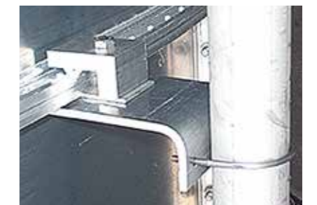
Typical J&D pipe support clip
