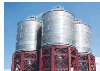
4 PTA Silos 3,450 m 3 for Korteks in Turkey (supplied via Zimmer)
