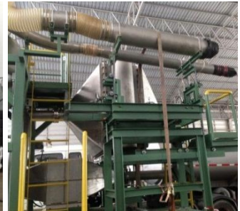
Mobile Sea Bulk Loading Station
